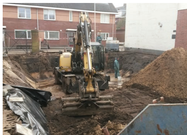
Ontgraving bronzone garage
